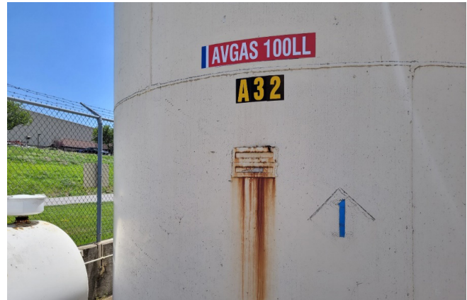
Figure A-7 Tank Typical Corroded Data Plate
