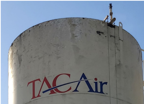
Figure A-6 Tank Typical Failed Coating and Corrosion
