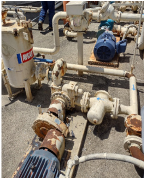
Figure A-11 Avgas Loading and Offloading System
