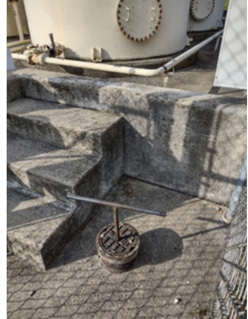
Figure A-13 Dike Area Drain Valve
