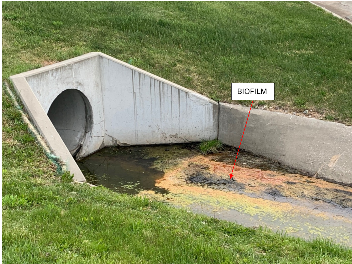
Figure 14: Biofilm Growth in Open Stormwater Channel Downstream of Monitoring Structure
