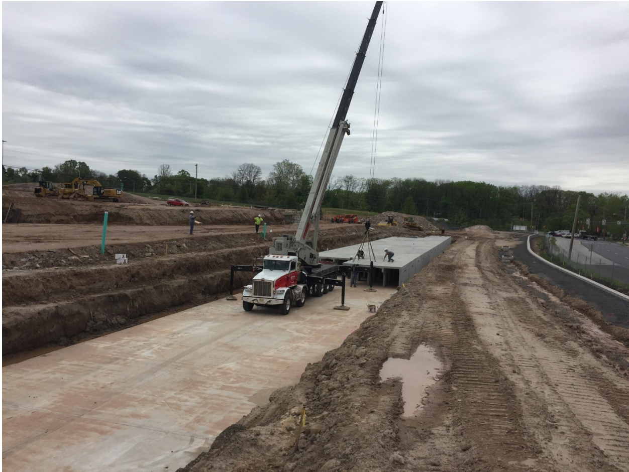
Figure 13: Example of Precast Concrete Detention Vault Assembly (Image Courtesy of StormTrap® Website)
